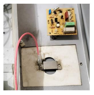
**6.** If original power box did have an internal air flow sensor, discard it and its wires associated with it. Find your 120v power source. The air cleaner needs to turn on and off with the blower. One option is to tap into blower power wire as 120v source. Second option, is to use general 120v current sensing relay to sense current on blower common wire. You can use Aprilaire relay 51.
